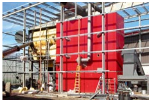
Installation of an 8,000 kW boiler
